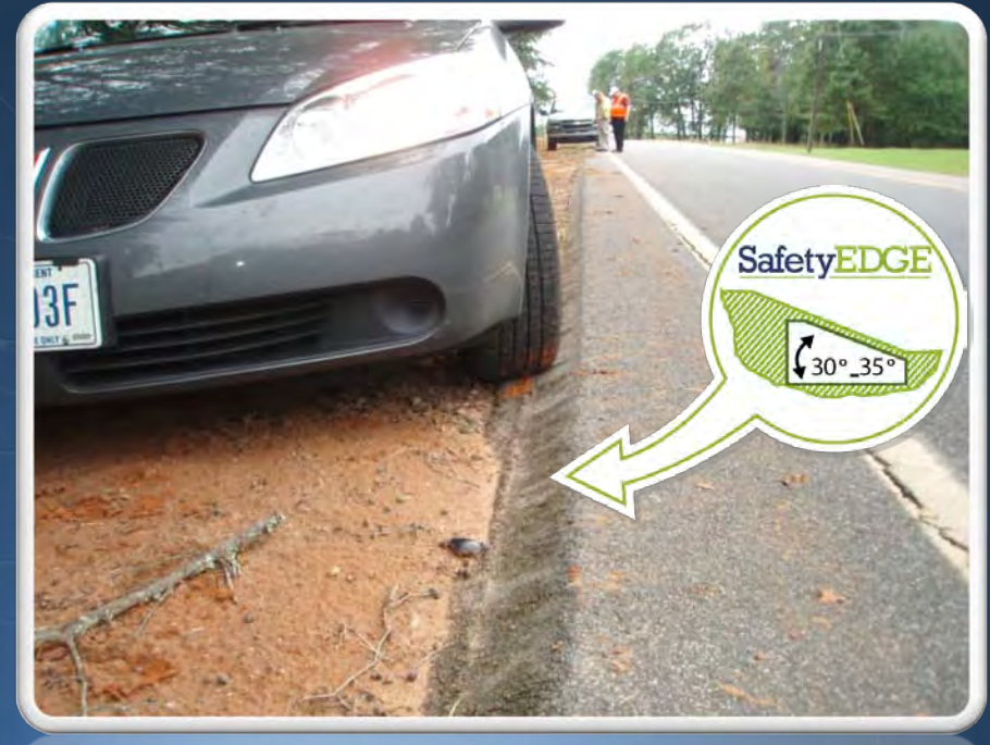
Paving with Safety Edge
