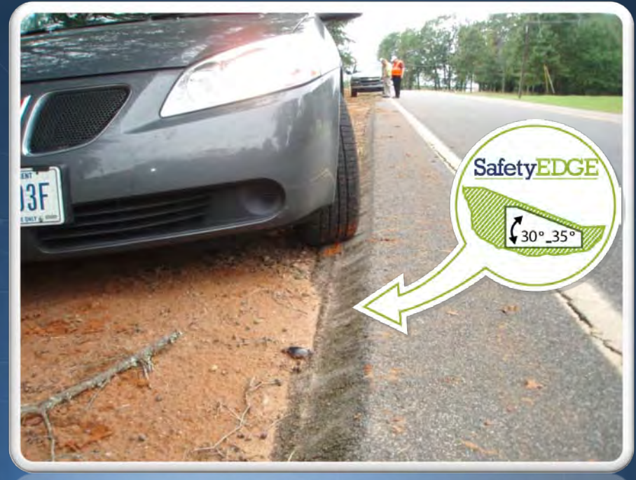
Paving with Safety Edge
