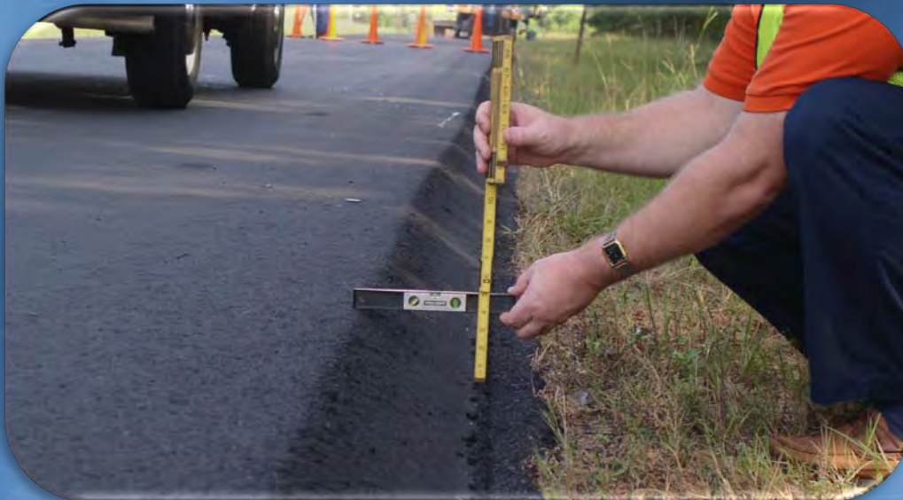
Asphalt Safety Edge Installation: Georgia
