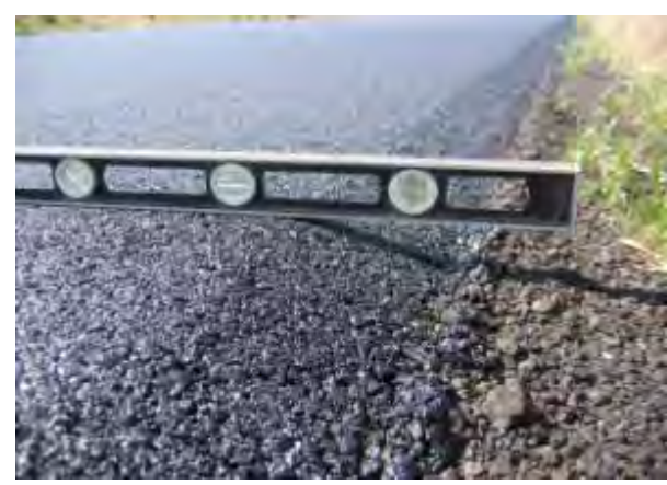
Figure 23. Angle of sloped pavement edge. Note the uniform compaction.
