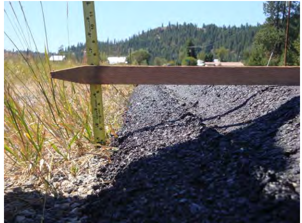
Figure 49. Close-up of edge treatment slope.
