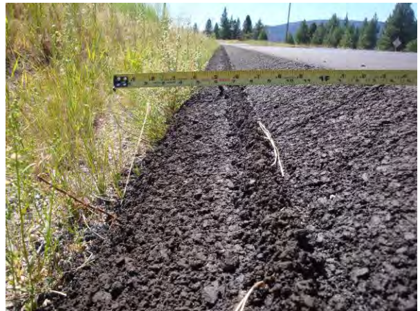
Figure 45. Close-up of edge treatment slope.
