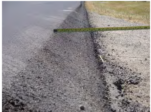
Figure 51. Closer view of slope of edge treatment.
