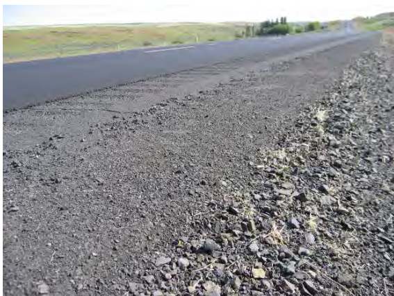
Figure 16. SR 395 before overlay. Note wide stable shoulder.
