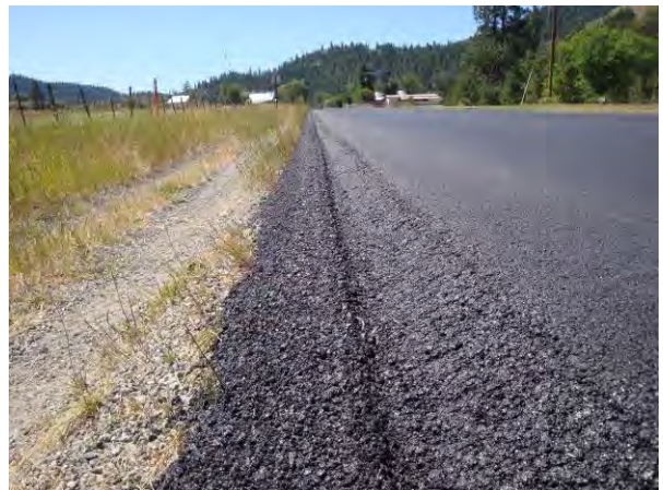
Figure 47. Another view of the edge treatment.
