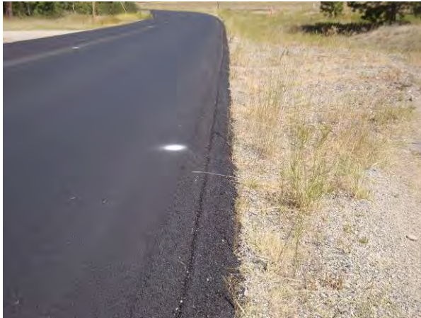
Figure 48. Edge treatment and shoulder area.
