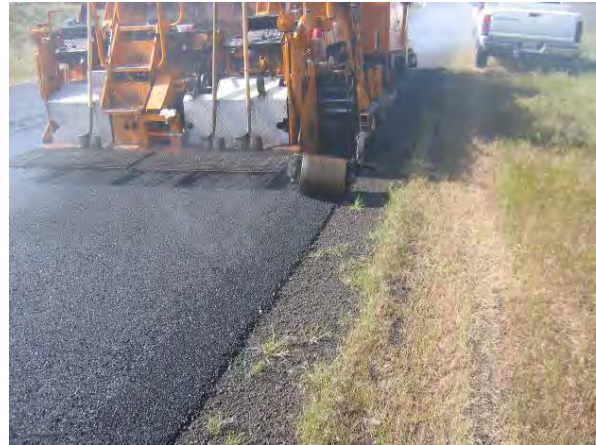
Figure 21. View of rolled pavement edge treatment.
