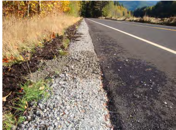
Figure 36. Shoulder material put back in place.
