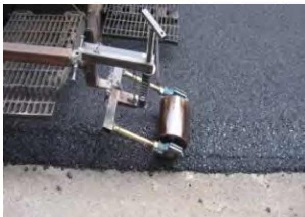
Figure 33. Roller added to compact the vertical edge at the top of the slope.
