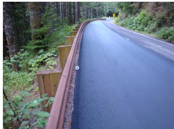
Figure 58. View showing uniform appearance of edge treatment.
