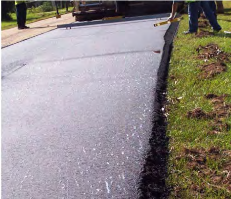
Figure 7. Pavement edge without the Safety Edge SM in foreground and with the Safety Edge SM in the background. (FHWA Safety Edge PowerPoint)
