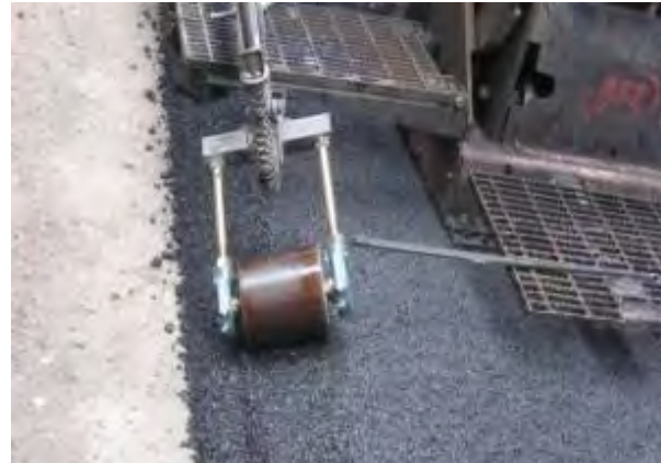
Figure 32. Roller added to compact the vertical edge at the top of the slope.
