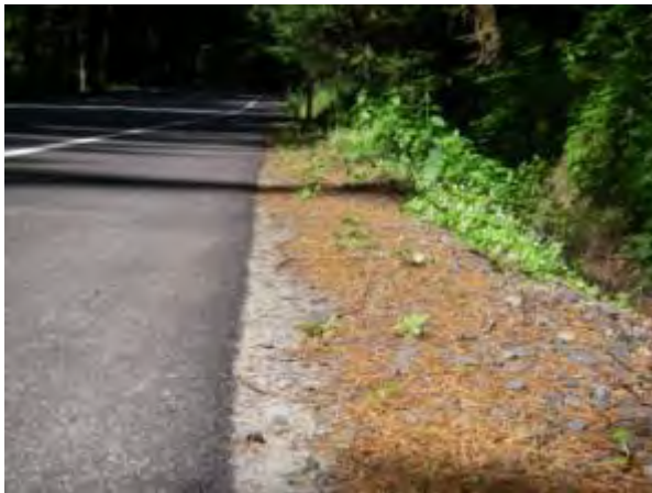
Figure 39. Another photo of the SR-410 pavement edge treatment one year after construction.
