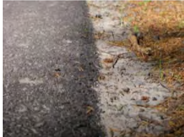
Figure 40. Close-up of pavement edge treatment on SR 410 one year after construction. Shows some exposure of pavement edge treatment.
