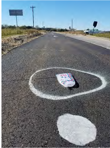
Figure 8 Typical asphalt test site
