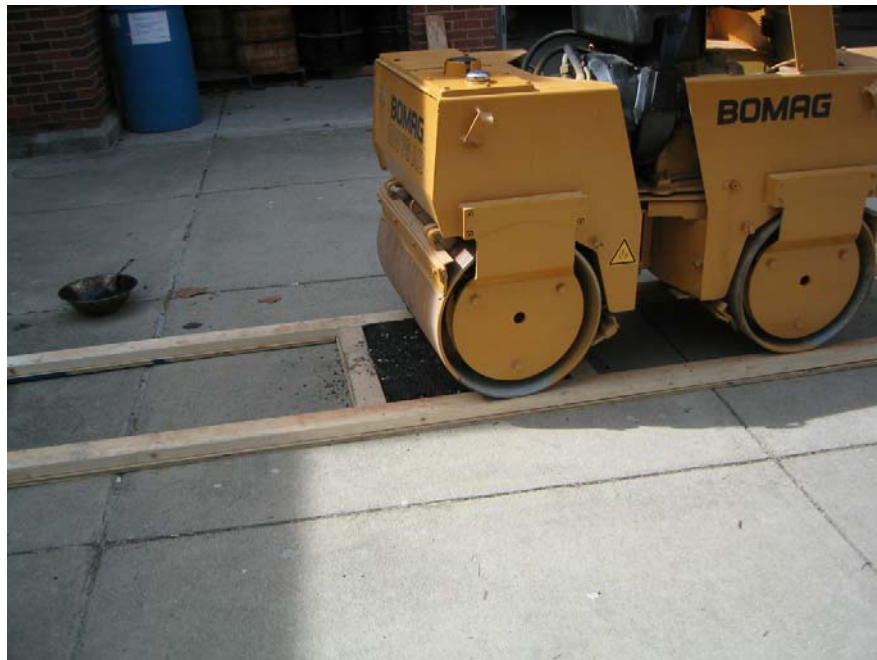
Figure 3. Compaction in Progress with 1.5 Ton Roller
