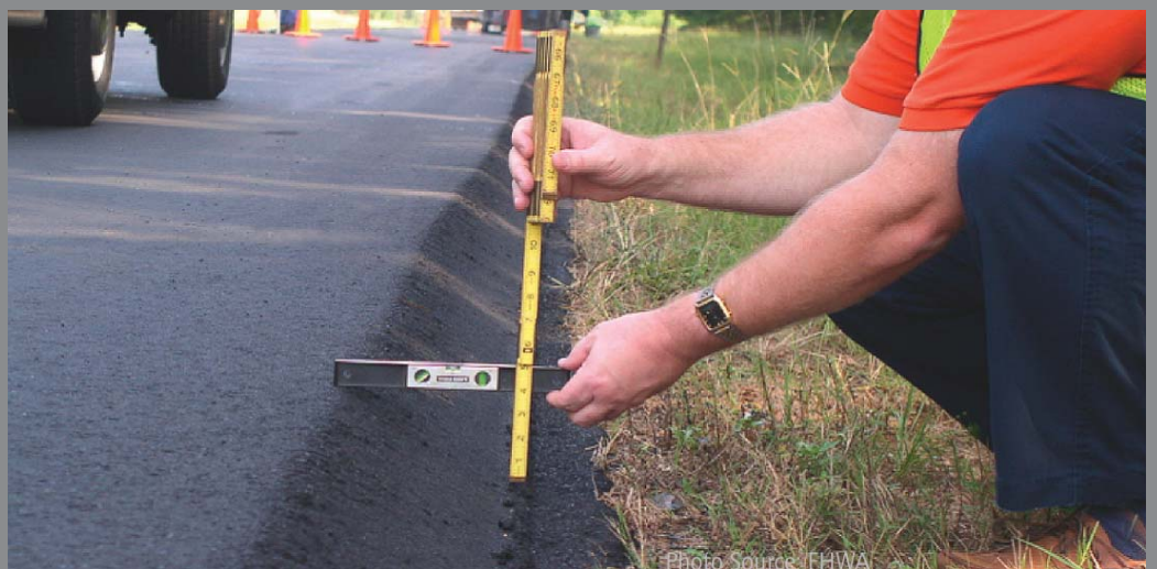
Photo Source: FHWA
