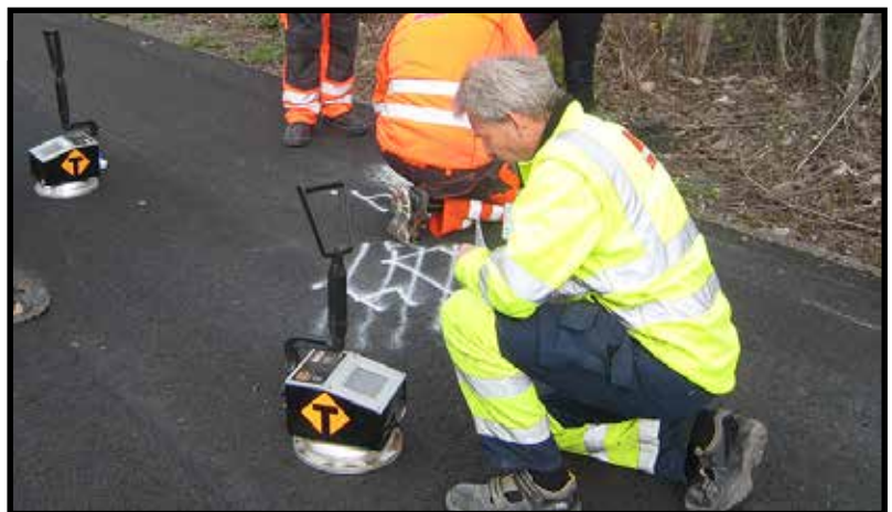
Veidekke AS and Statens Vegvesen testing PQI 380 asphalt density gauges.
