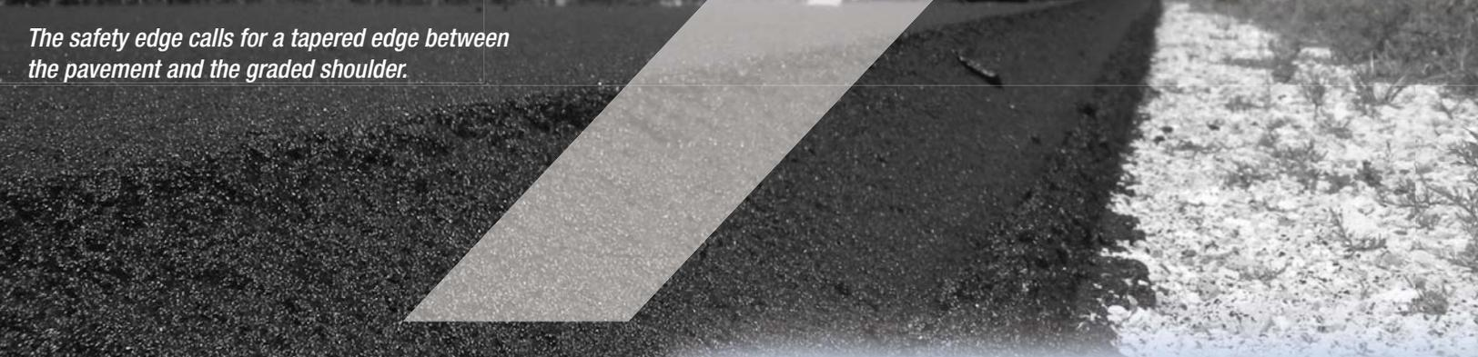
*The safety edge calls for a tapered edge between the pavement and the graded shoulder.*
